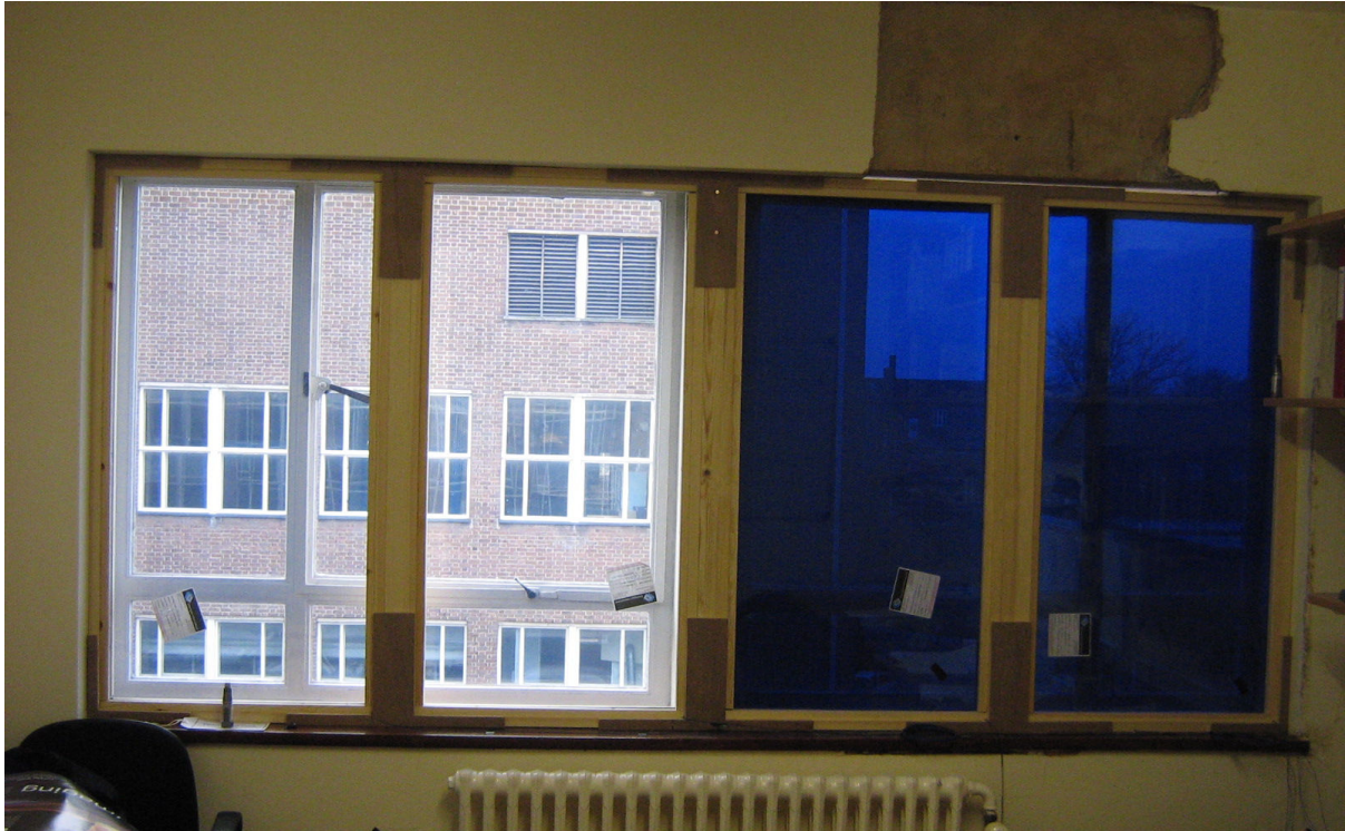
Figure.4d shows two of the SPD windows switched on, while the other windows are still unconnected
