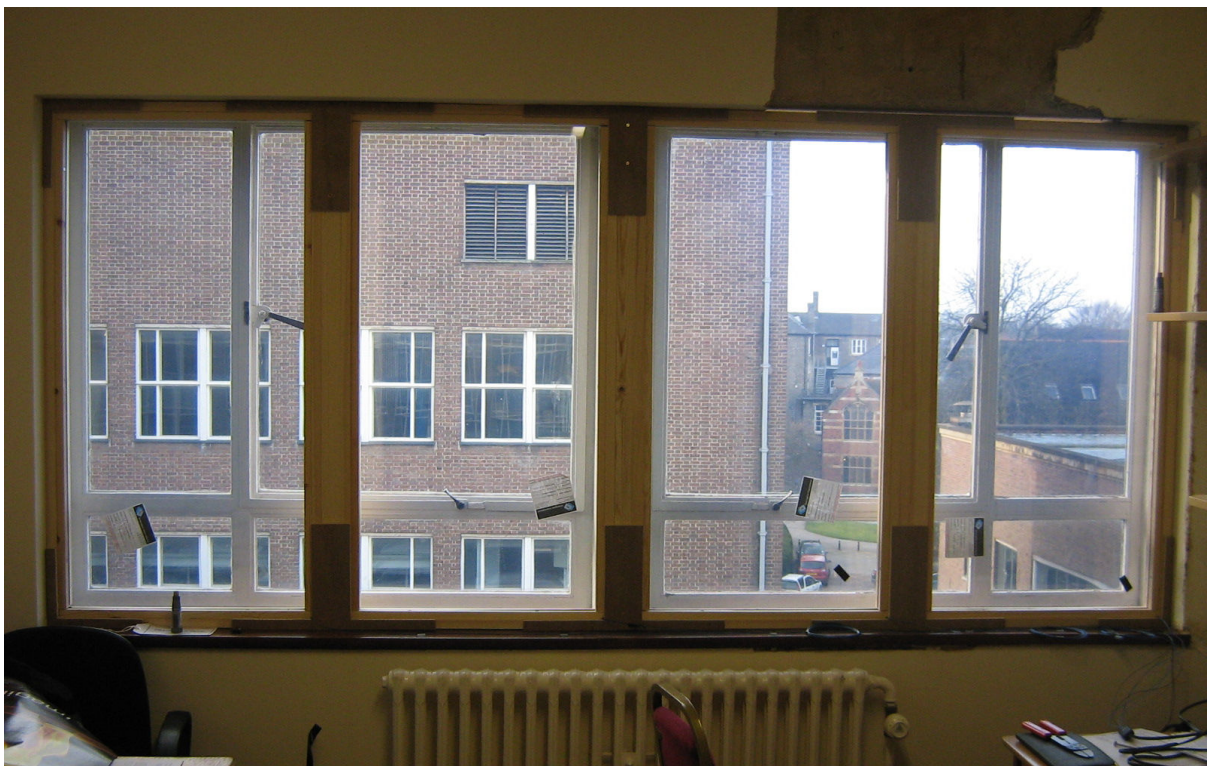
Figure.4e shows all the SPD windows connected and switched on. The windows display a clear state without the blue tint previously shown.
