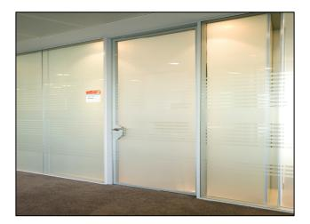
All LC SmartGlass panels are bespoke manufactured using a lamination process which encapsulates a PDLC film between 2 or more glass sheets. Using a minute electrical current, users can immediately switch the LC SmartGlass from clear to private (opaque) and vice versa.
